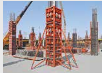
Column Formwork
