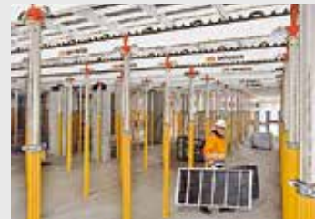
Slab Formwork
