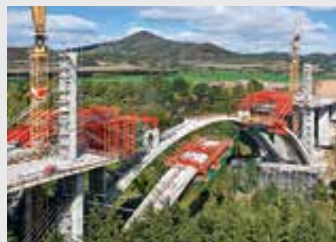
Bridge Formwork
