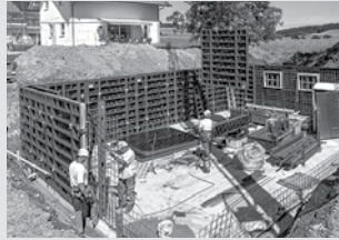
Wall Formwork
